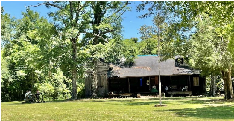
The Cabin at Camp Pushmataha is located at the Citronelle Surrender site.
